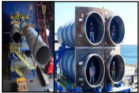
Integrated Tube / Hull Construction
